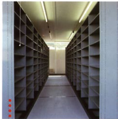
6 Shelving completed and awaiting end panels and drive wheels
