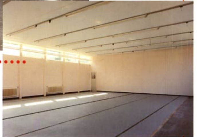
2 Rails are laid out and levelled to 1 in 1000. Once levelled, grout is applied and cured before taking load
