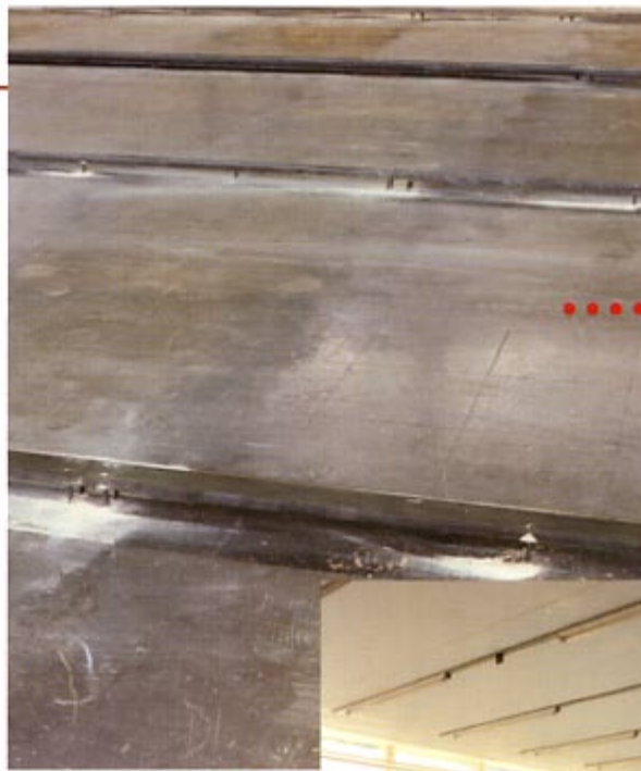
3 The infill floor is built up to the level of the rails ready to receive storage equipment
